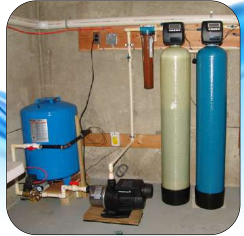
Softener & Pressure Booster Systems
